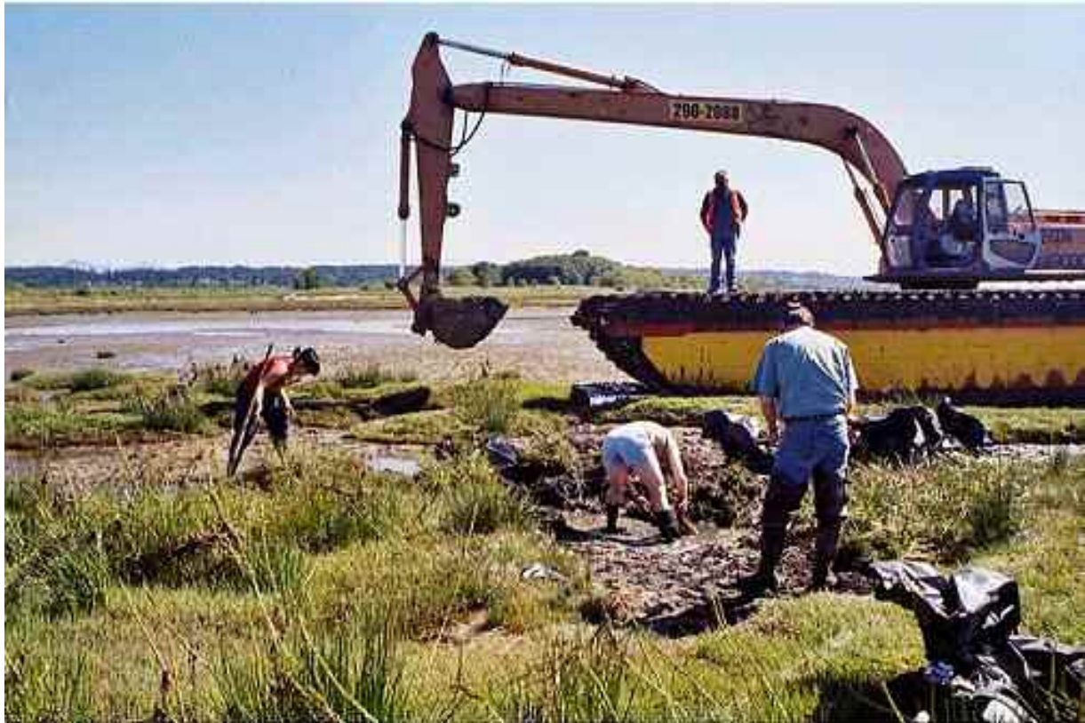
Figure 5. Spartina Removal Methods (Excavator & Manual Removal)
